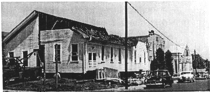
Disassembling the original building
