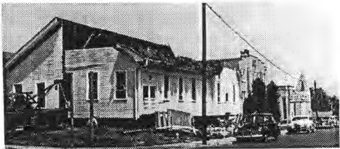
Disassembling the original building
